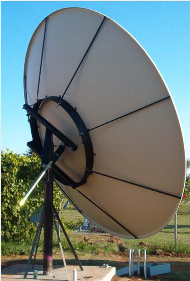
**Sectional antennas must be handled with care not to twist or distort sections while handling for installation.**
