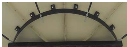
Figure #7 Back Brace To Clip
